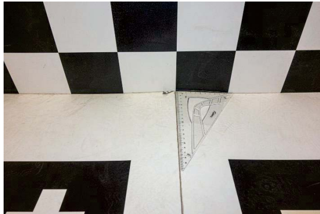
Finding a line perpendicular to the wall
