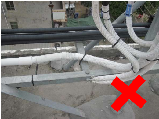
Multiply the grounding point
