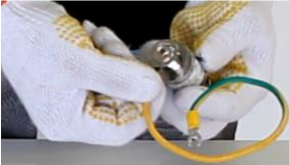
Figure 4-3 Connect the Ground Wire of GPS Lightning Arrestor
