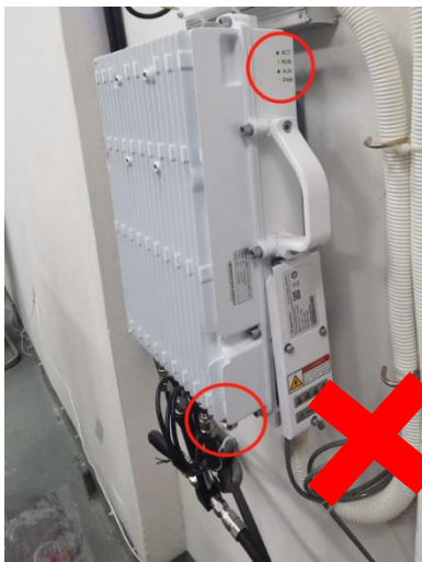
The RF feed system does not connect, the cell is activated and RF transmits signal
