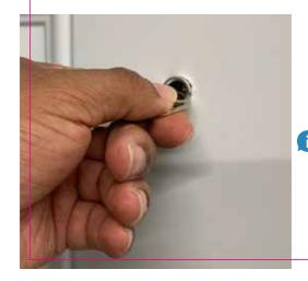
You may have to secure the outdoor side of the peephole while unscrewing the indoor portion to keep it from spinning.
