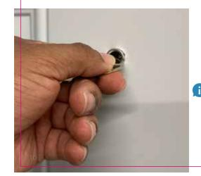
You may have to secure the outdoor side of the peephole while unscrewing the indoor portion to keep it from spinning.
