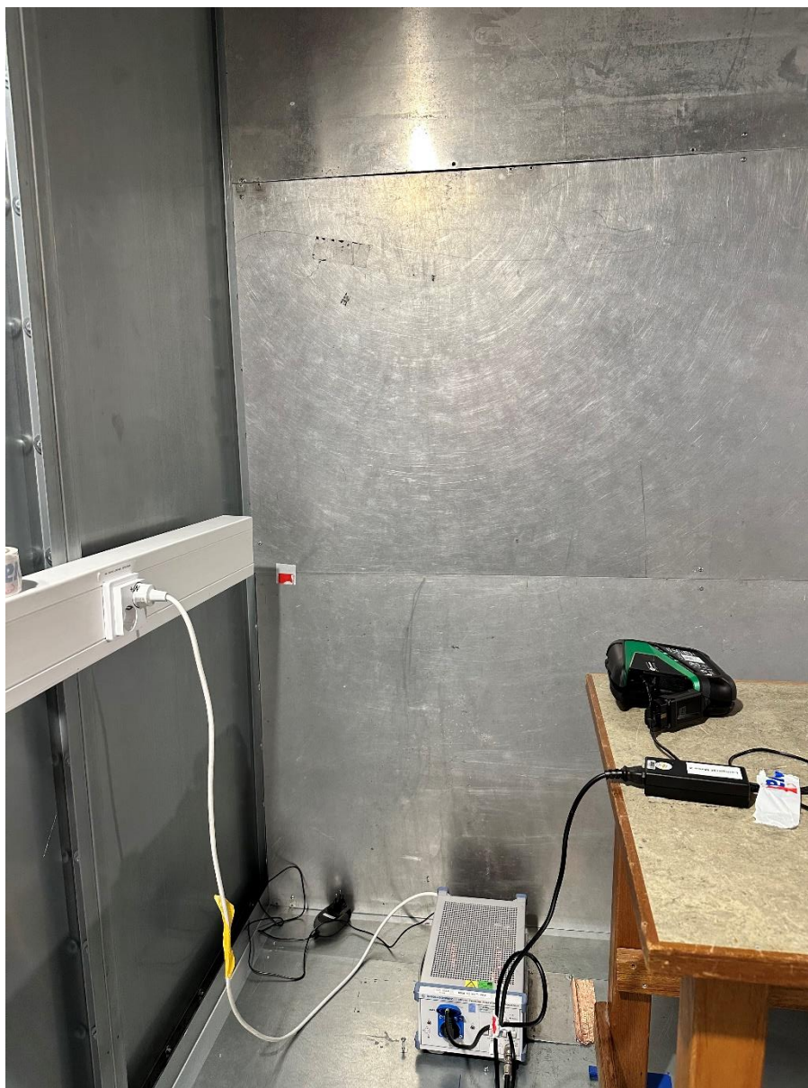
Photo 6: Photographs AC Power Line conducted emission
