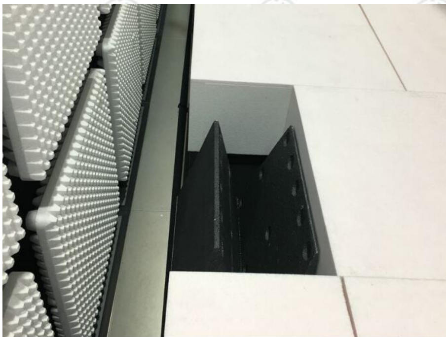
There are absorbing materials under the ground
