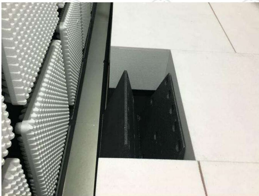
There are absorbing materials under the ground
