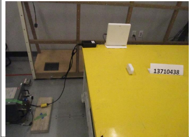
AC LINE FRONT PHOTO
