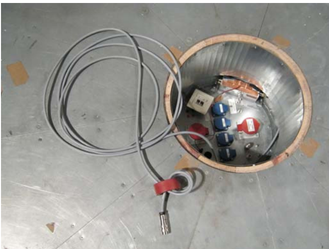
Photograph 2.3-3: Junction box with signal and supply cable and ferrite connected
