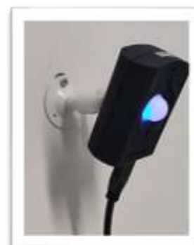
Image 11: wall mount installed
