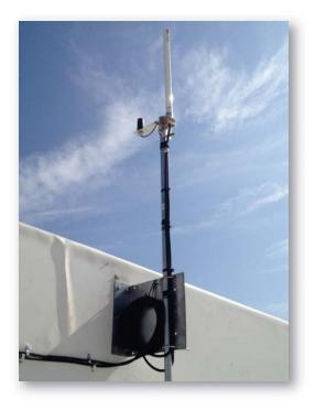
Antenna mounted on 12" wall mount "L" bracket with a 1.5" pipe extension so the antenna clears all obstructions above the roof line.
