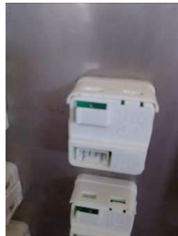
Figure 3-1-2 Elevator push-button back
