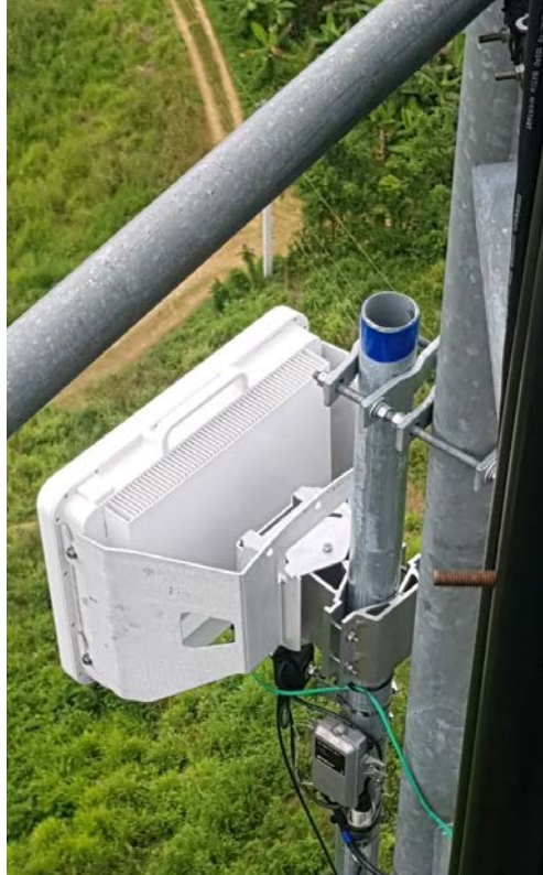
BN Installed on Tower
