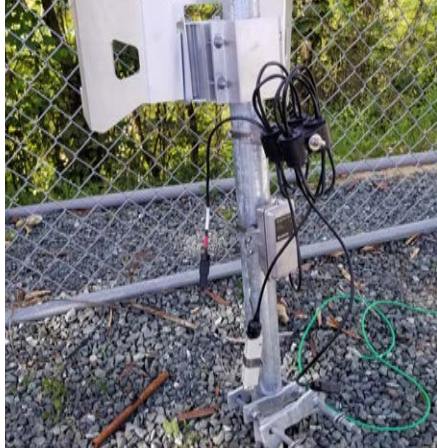
Outrigger installed with BN Mount
