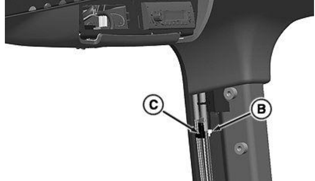
Antenna Coaxial Cable And Business Band Radio Power/Ground Plug Coiled Behind Right Rear Corner Post Cover
