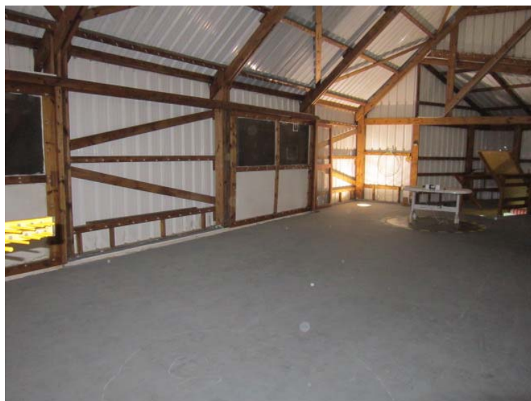
Photograph 8.2.3 Setup for final radiated emission measurements
