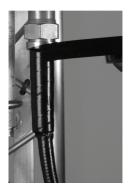
Cut a piece of butyl rubber large enough to wrap around the connector and extended past the first layer of tape, stretching it so that it will wrap completely around the connector and cable. Press the rubber against the connection and cable, ensuring there are no gaps at the edges.
