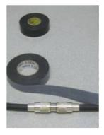
2. Peel back a length of the protective barrier and trim off if needed. Minimize contact with the surface to ensure proper adhesion.
