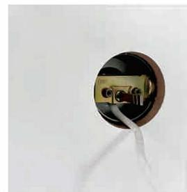
The connecting wire must pass under the lock body
