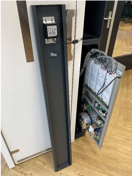
Barcode reader in front panel and open electrowall with transformer, ballasts, sensor PCB and on/off switch.
