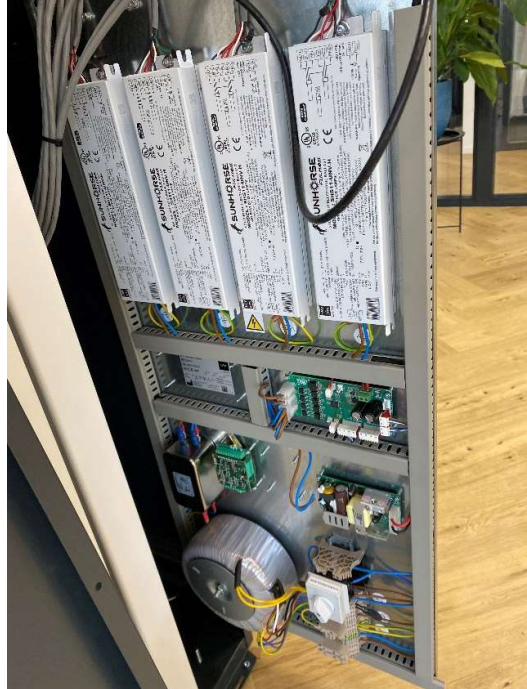
Barcode reader in front panel and open electrowall with transformer, ballasts, sensor PCB and on/off switch.
