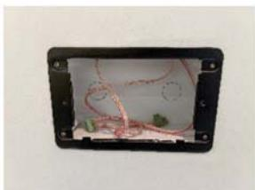
Fix the metal bracket on back box with 4 screws.
