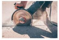
5.Put the mounting bracket on stone or cement surface, cut the mounting bracket along the dot line with grinder if you don't have enough installation room, which is only for your reference, cutting varies based on your actual application
