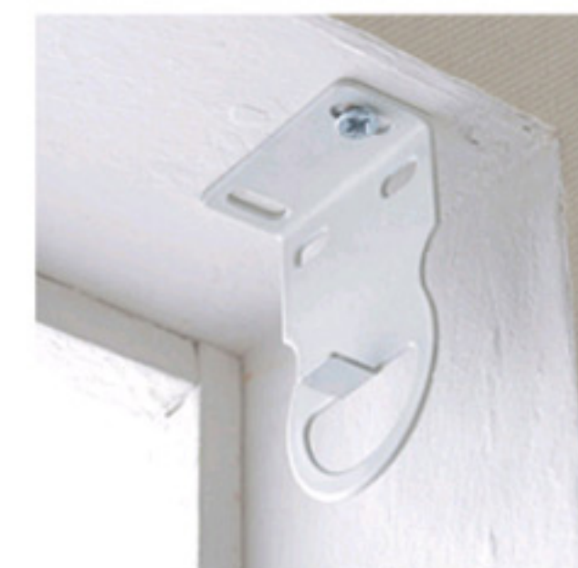
Install screws and bracket
