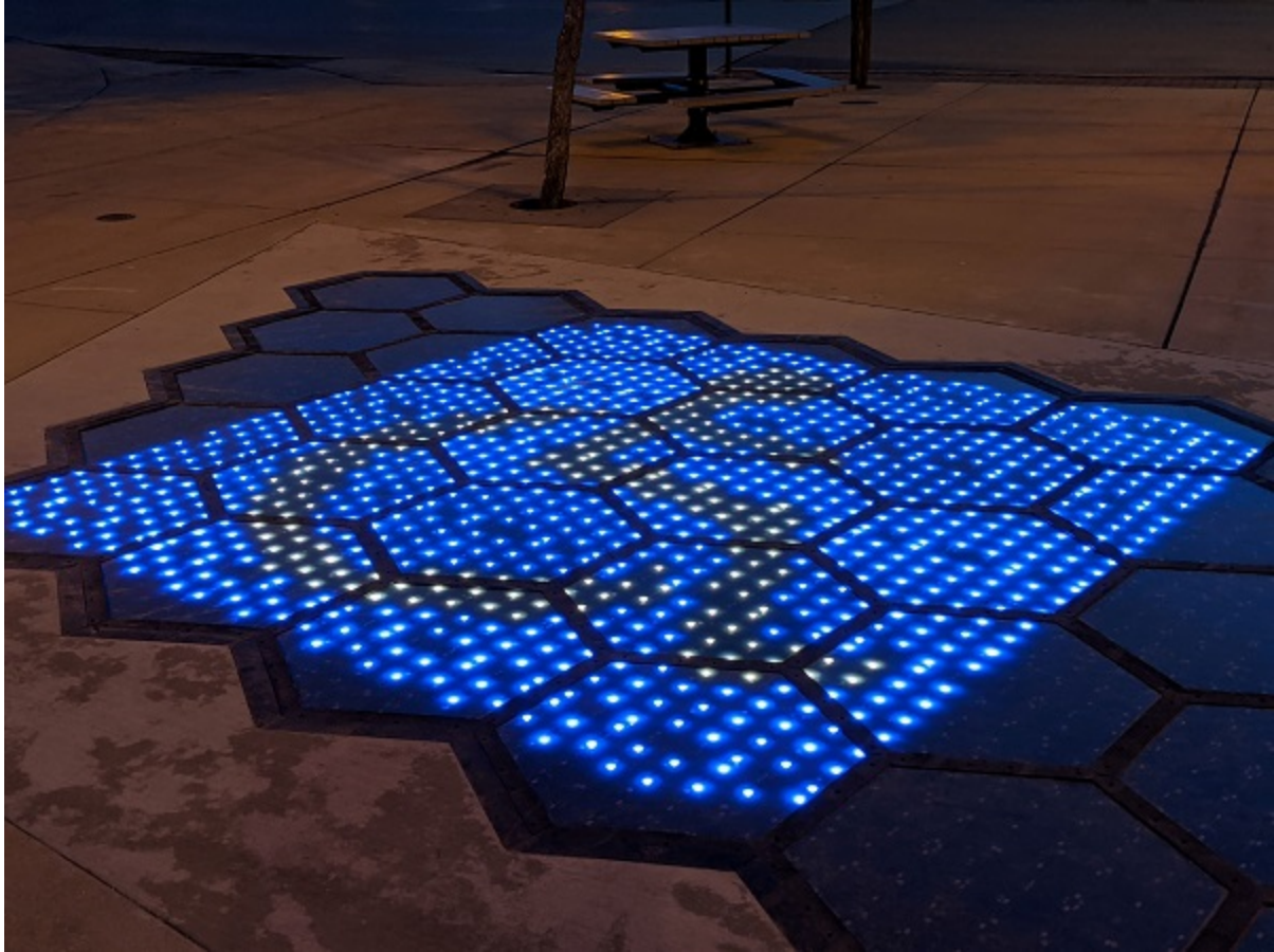
Figure 9. Photo. Actual Sandpoint, Idaho 30-panel installation showing handicapped pattern.
