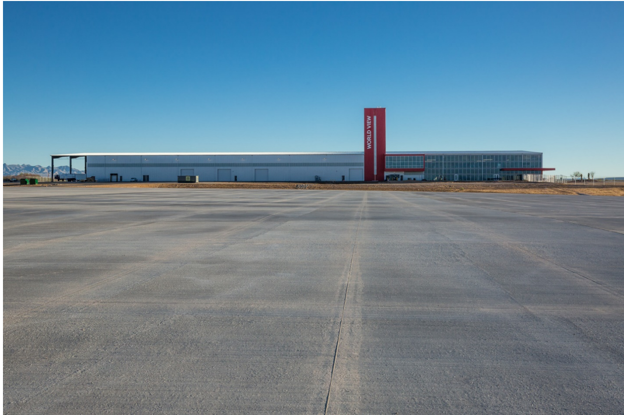
Figure 2. Spaceport Tucson & World View's Facility
