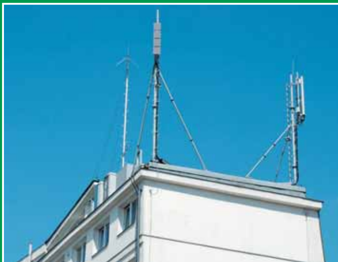
TETRACUBE panel antenna length around 1.5 meters, 12 Kg (only antennas; mast not included)
