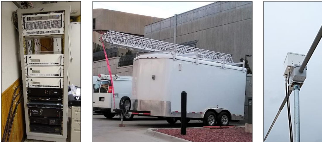
Figure 1. The radar's rack, specialized trailer with 33-m telescopic tower, and one of the receiving antenna assemblies.
