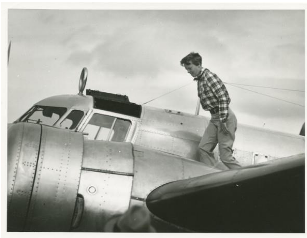
Amelia Earhart's L-10E showing the DF Loop and Transmit "V" Wire Antenna
