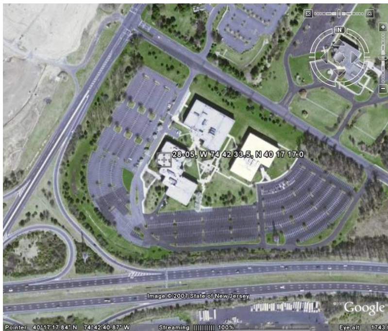
Figure 2. Aerial View, Site #1
