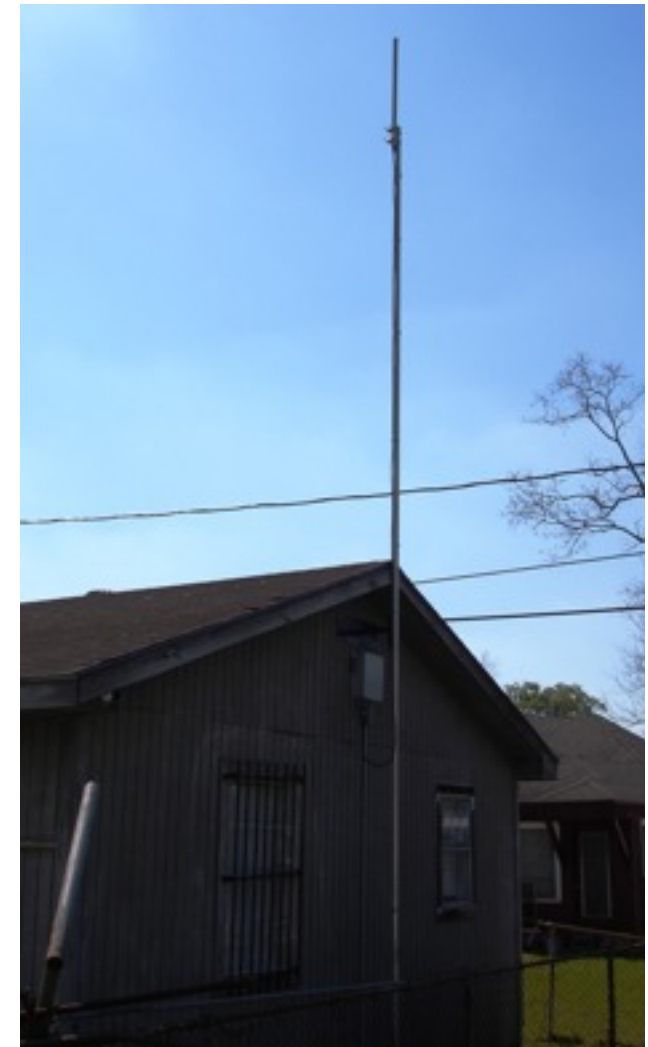
Existing monopole WiFi antennas - compliant with City of Houston Ordinances and installed by professional installers
