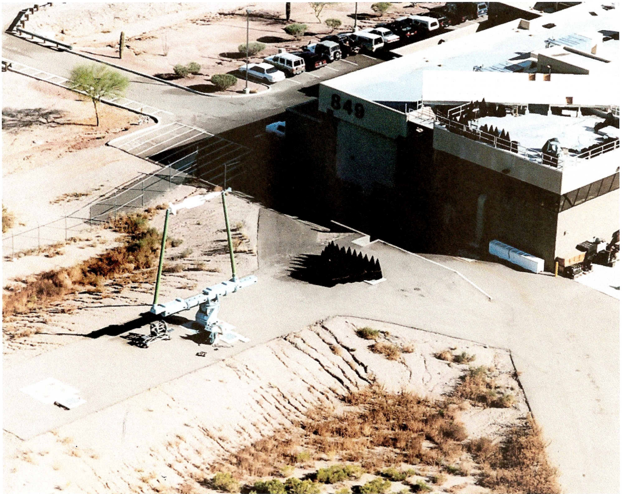
Figure 2. The scatter fence diffuses the RF energy in many directions, reducing the potential for interference.
