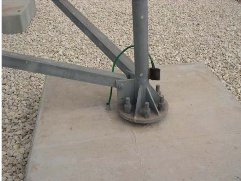
Tower grounding example
