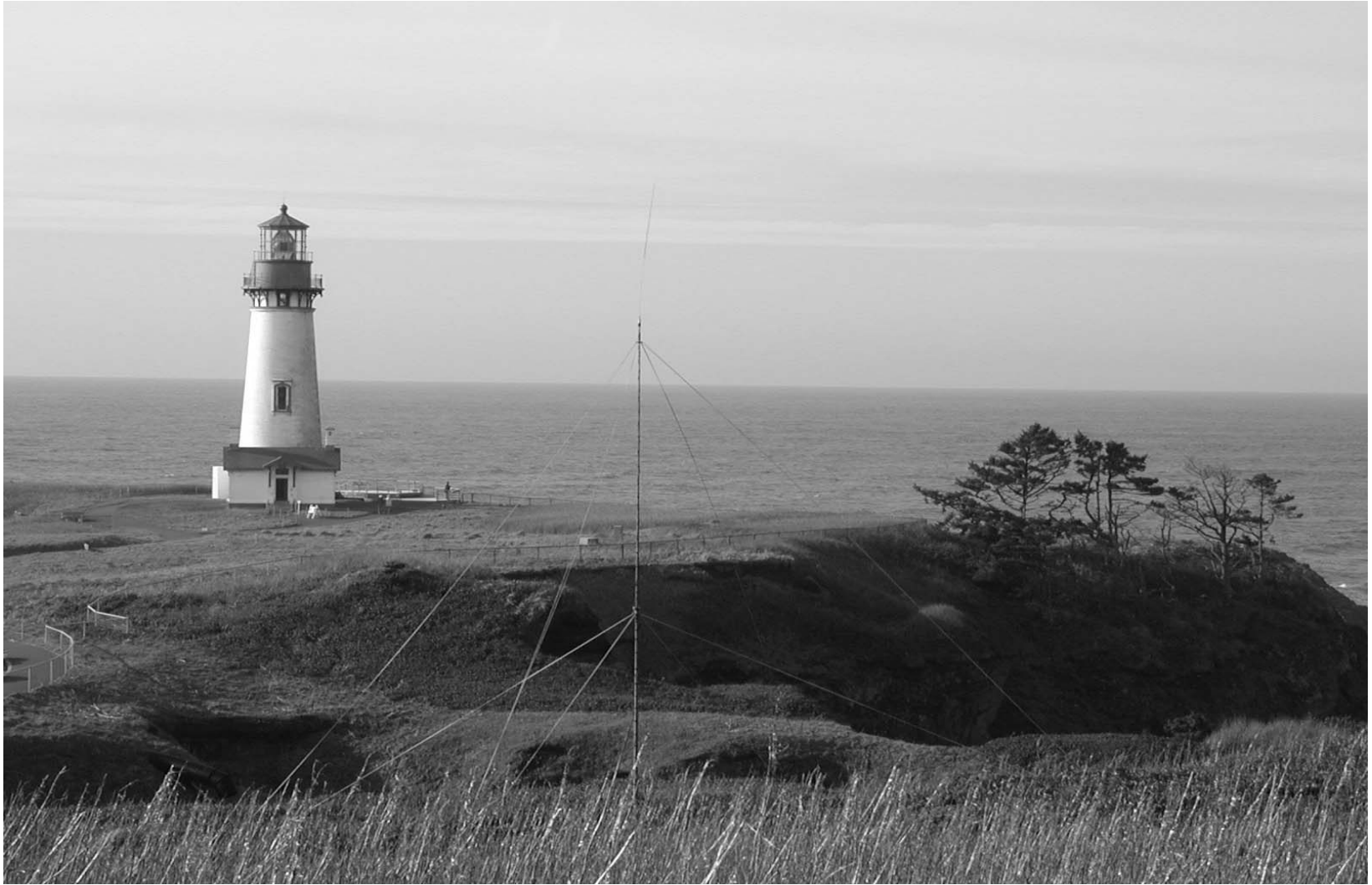
Photo: showing 12m (vertical height) transmit antenna.
