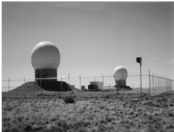
Figure 3-5 - The Radomes of a GES
