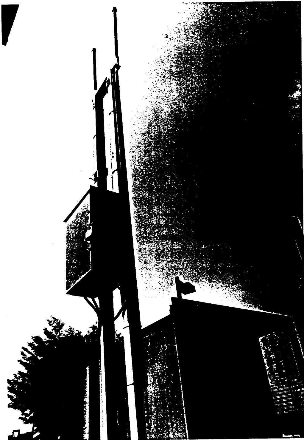
Public Microcell Installation No. 1 Silver Spring, Maryland Figure 3.2-2
