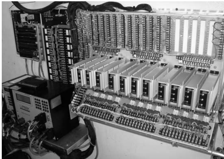
The picture below shows the control devices that operate the traffic lights around the Plaza Las Americas Area
