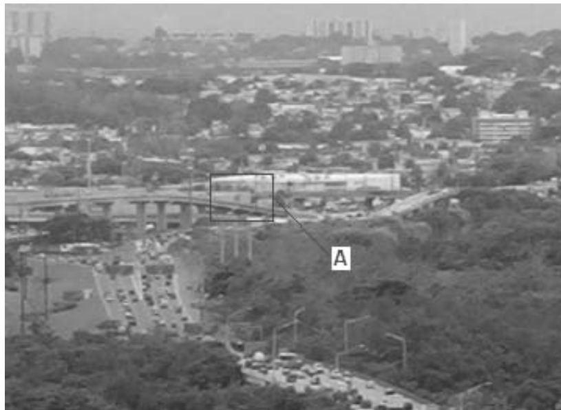
A. Lighting Pole where the Antenna will be placed.
