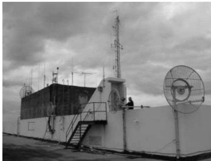
The picture below shows the roof top of Minillas Sur Building
