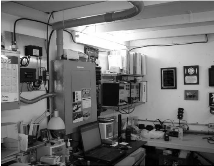
The picture below shows the control devices that operate the traffic lights around the Plaza Las Americas Area
