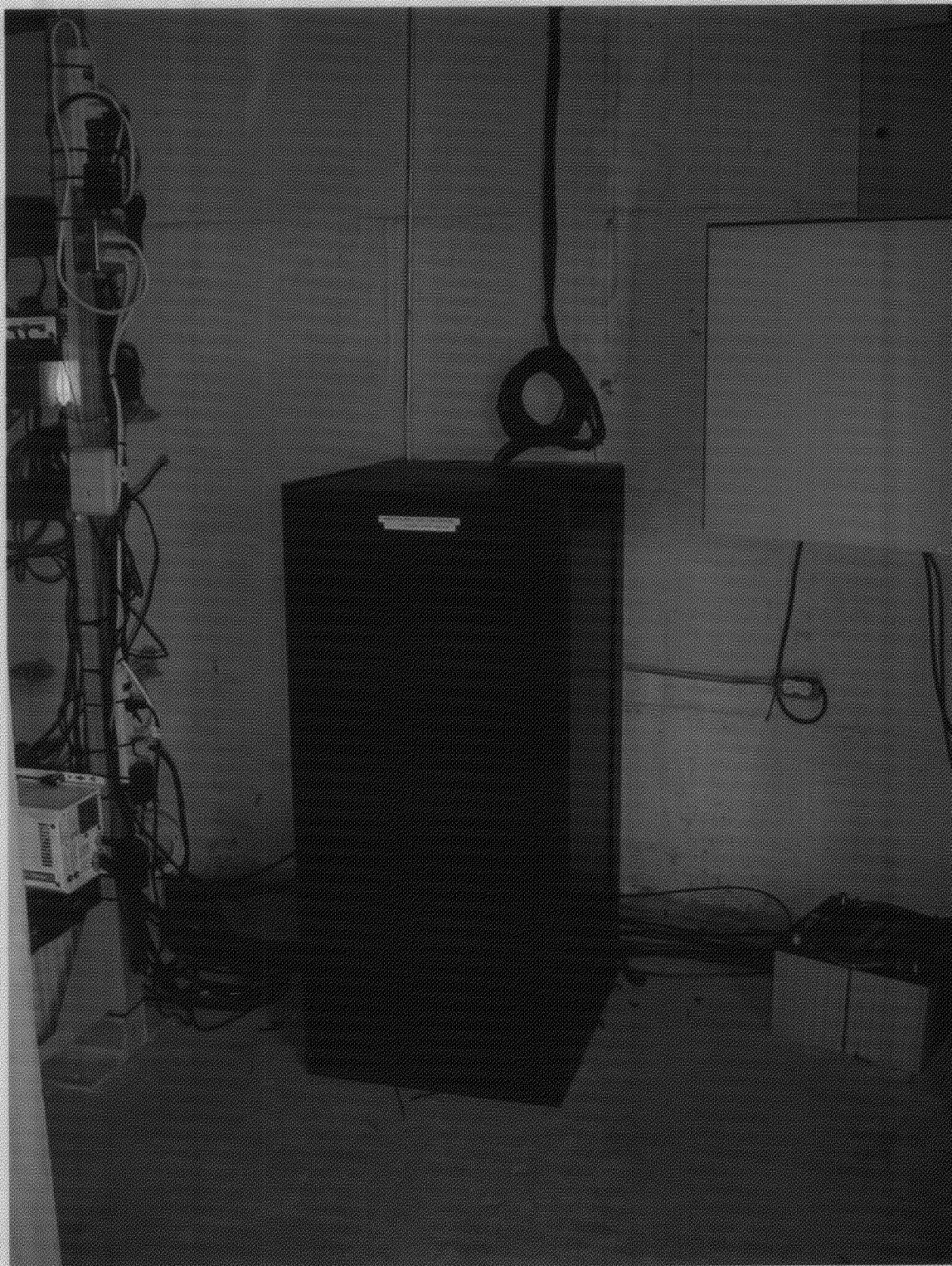
Figure 11 – Neptuneo equipment cabinet.
