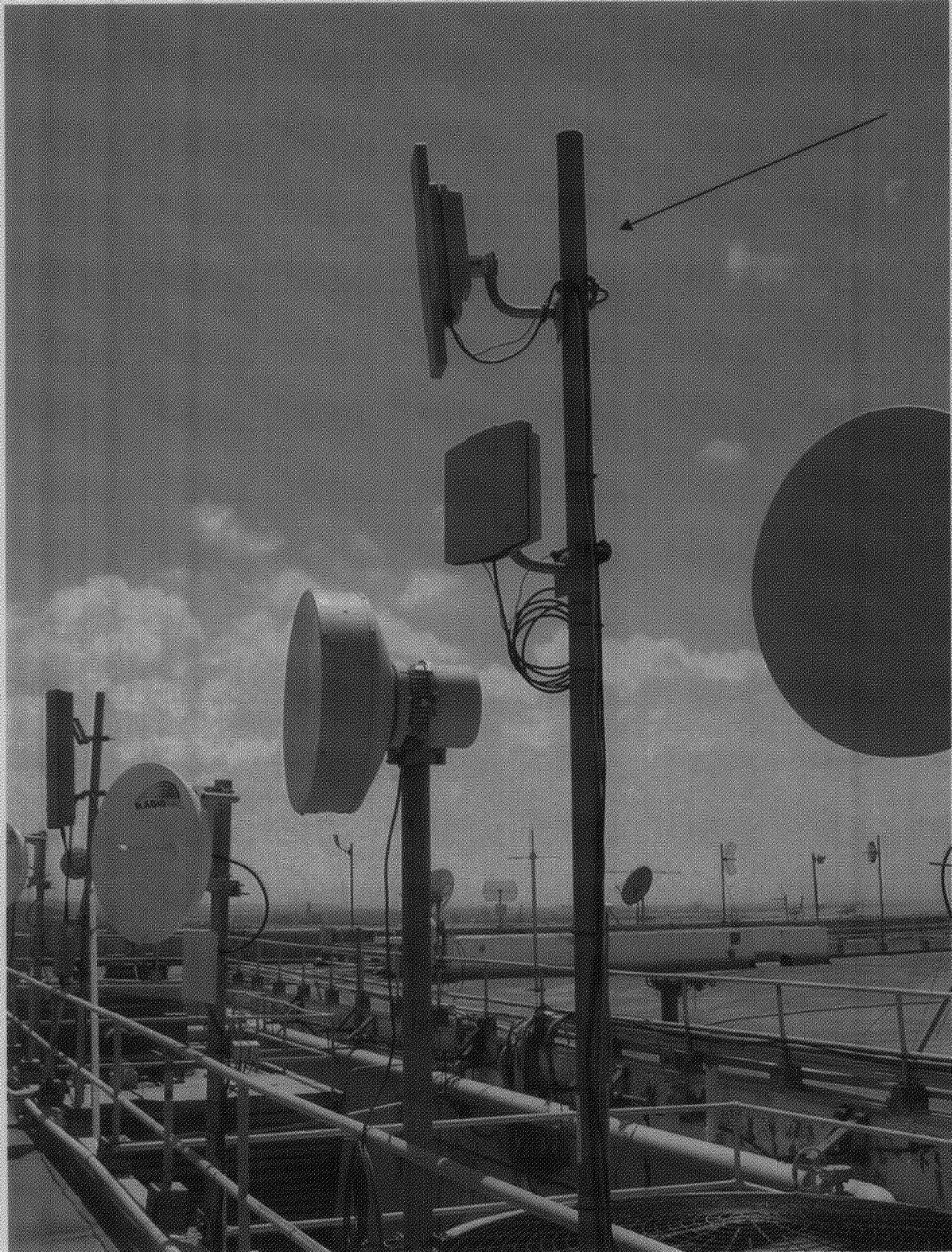
Figure 10 – Mast #3 with NEP6 and NEP7 emitters.
