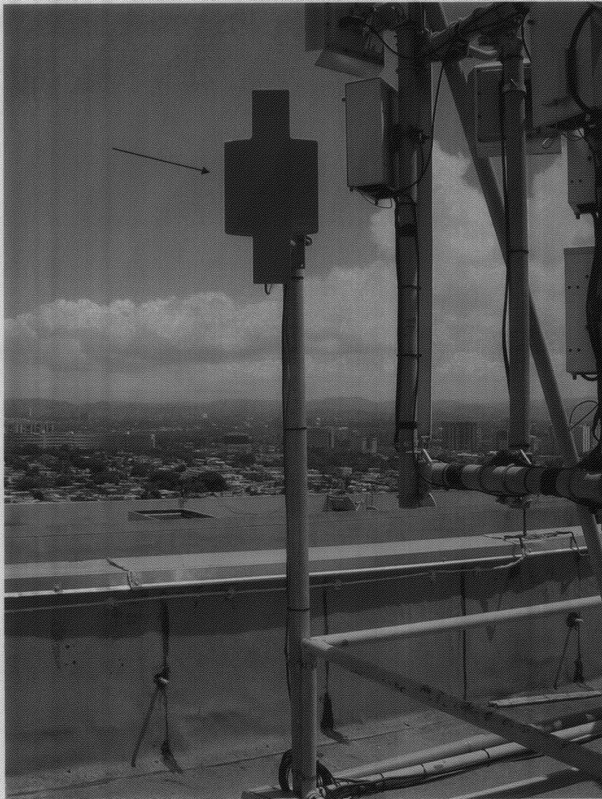
Figure 7 – Mast #2 with NEP5 emitter.
