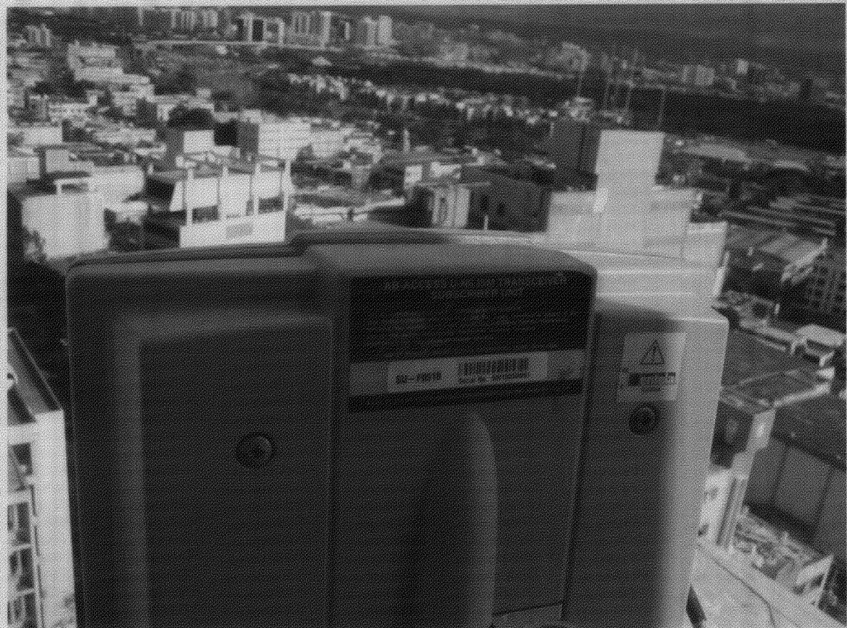
Photo 3 – Back of Apparent Neptuno Networks Antenna at Site 2
