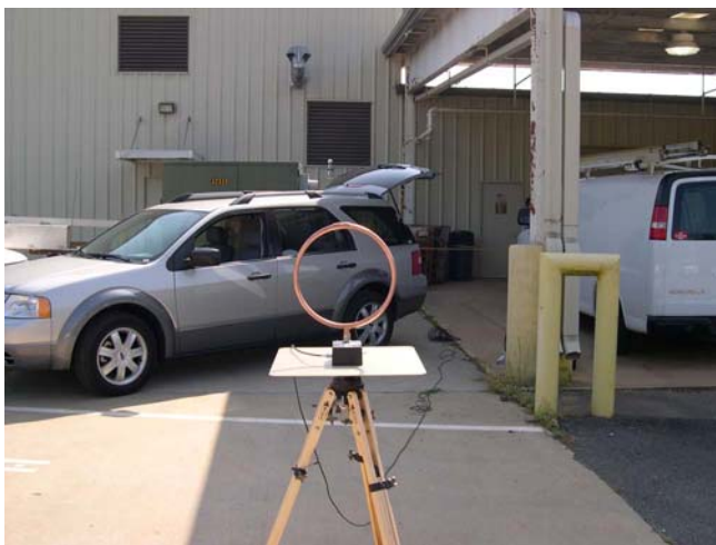
JEMC Location - Pad Mount Transformer
