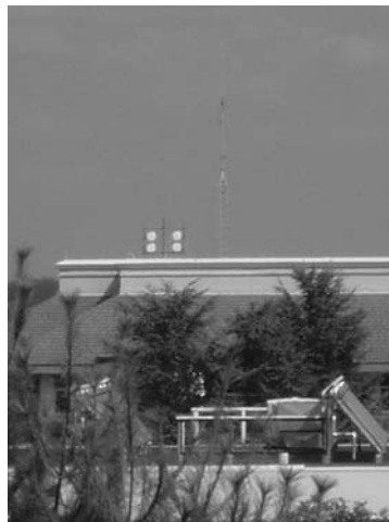
Figure 3 - Site 6 (Montgomery College Roof)
