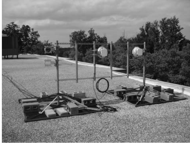
Figure 2 - Site 2 (GTEC Roof)
