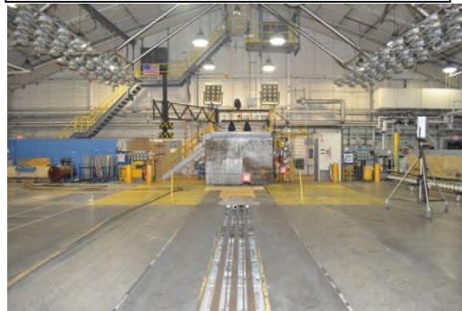
Figure 8 – Inside MPG Crash Test Building Facing North
