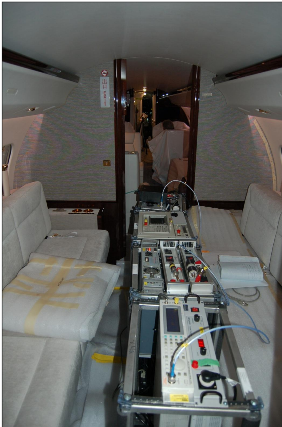
Photo 2: Typical Generator Drive to Amplifiers
