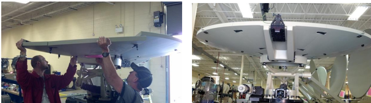
Figure 24b & 24c. Attachment of Panels 4, 5, and 6
