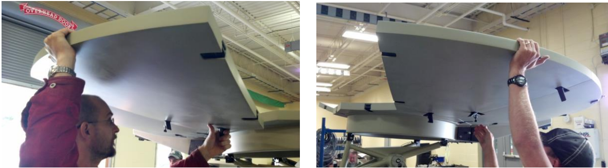
Figure 23b & 23c. Attachment of Reflector Panels 3 and 7
