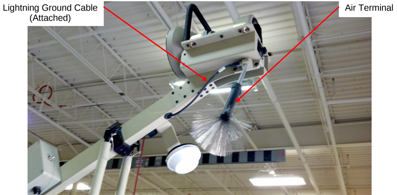
Figure 32. Attaching the Lightning Air Terminal
