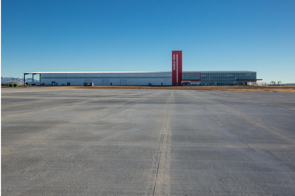
Figure 2. Spaceport Tucson & World View's Facility
