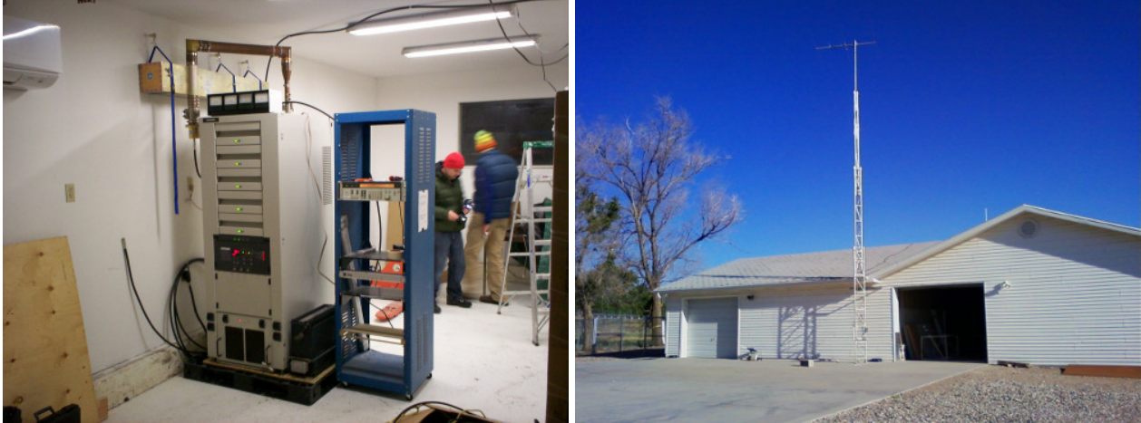
Figure 2: Station WF2XHR, broadcasting a 54.1 MHz carrier wave at 2 kW from Delta, Utah. Left: “Low” power analog TV transmitter as installed in the Millard County Cosmic Ray Center. Right: Outdoor view of Cosmic Ray Center with mast and 6-element Yagi antenna. Work on this transmitter station was completed January 2011, just prior to submission of this proposal.
