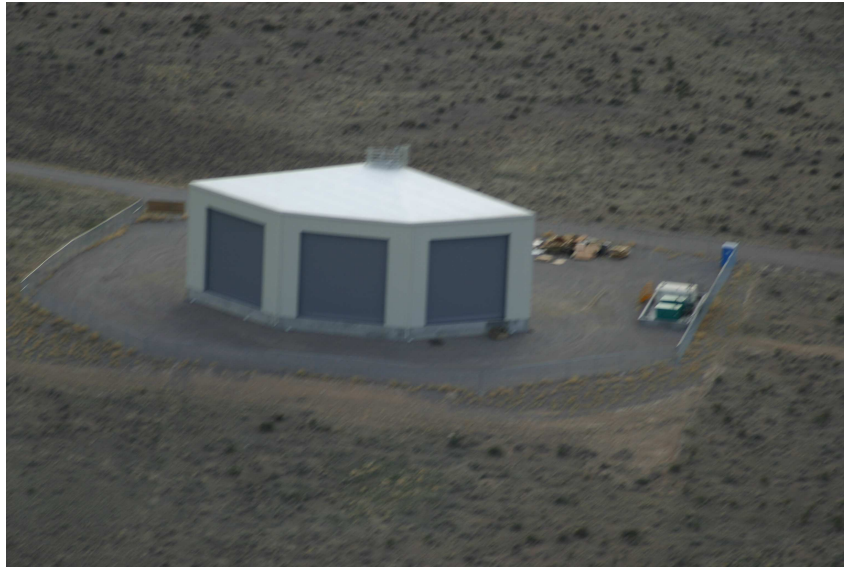
Figure 8: Long Ridge fluorescence detector facility as seen from the air. The command center was not built at the time this photo was taken. Note the green five feet tall diesel generators on the right.
