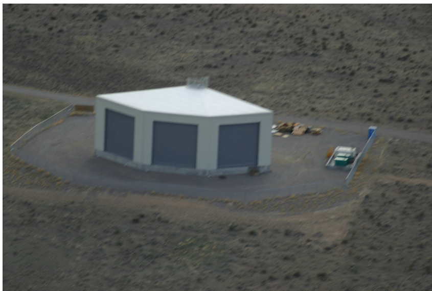
Figure 8: Long Ridge fluorescence detector facility as seen from the air. The command center was not built at the time this photo was taken. Note the green five feet tall diesel generators on the right.
