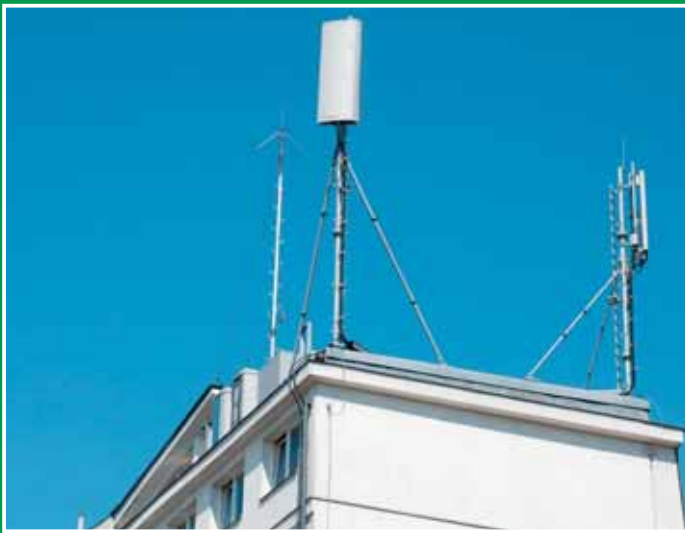
Traditional tetra panel antenna length around 2 meters, 22 Kg (only antenna, mast not included)
