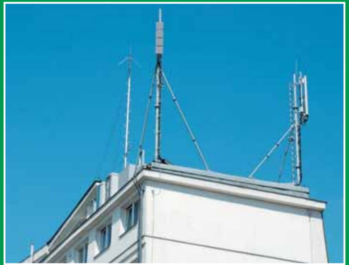
TETRACUBE panel antenna length around 1.5 meters, 12 Kg (only antennas; mast not included)
